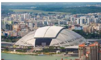
Gambar 12. National Stadium Singapura
