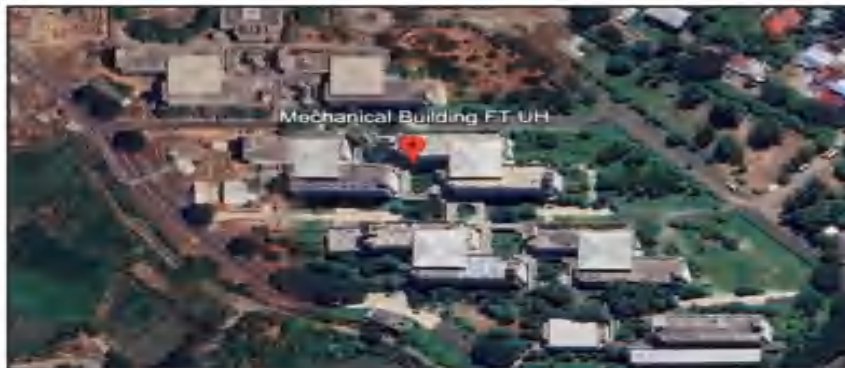
Gambar 10. Mechanical Building Ft-Uh
