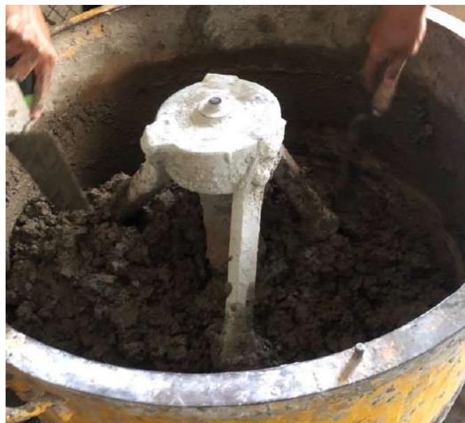
Gambar 8. Proses Mixer Campuran Beton
