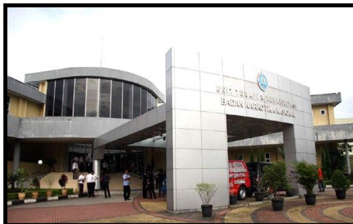
Gambar 23. Front view main entrance
