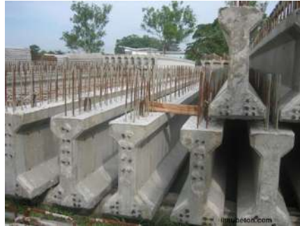
Gambar 5 Beton Pra Tegang
