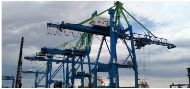
Gambar 2.1 Ship to Shore (STS) Crane / Container Crane
