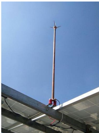
Gambar 2 4 Lightning Arrester
