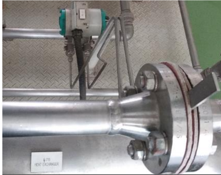
Gambar 2.10 Orifice D/P Transmitter
