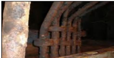
**Gambar 4.** *Uniform corrosion*
