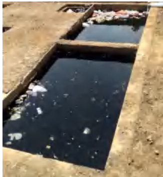
(a) Inlet Kolam Pengolahan Air Lindi
