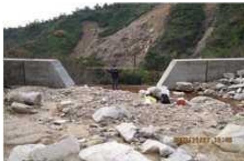
Gambar 1 Check dam Tipe Tertutup (Sumber: Maricar and Lopa, 2013)
