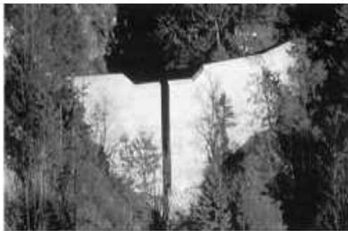
Gambar 3. Check dam tipe slit (Sumber: Armanini and Larcher, 2001)
