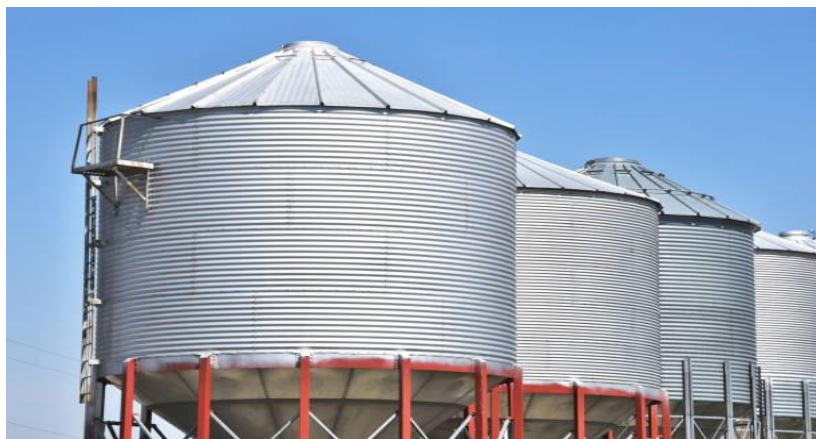
Gambar 10. Cone Roof Tank
