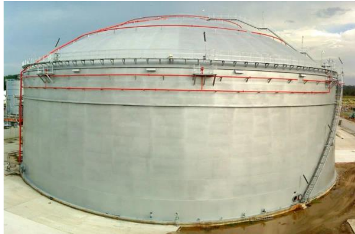
Gambar 11. Tangki Fixed Dome Roof
