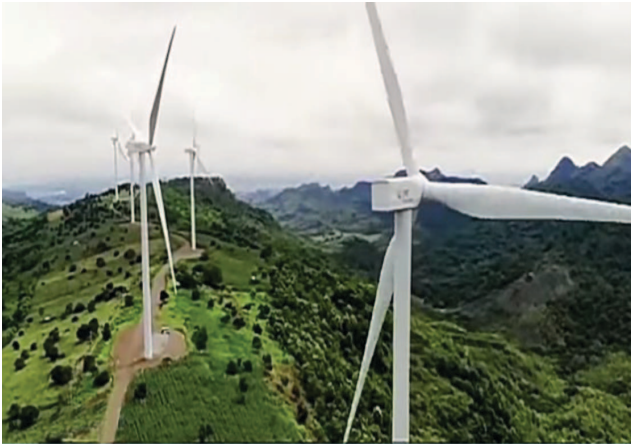
Fig. 2. Sidrap Wind Turbine with a capacity of 75 MW
