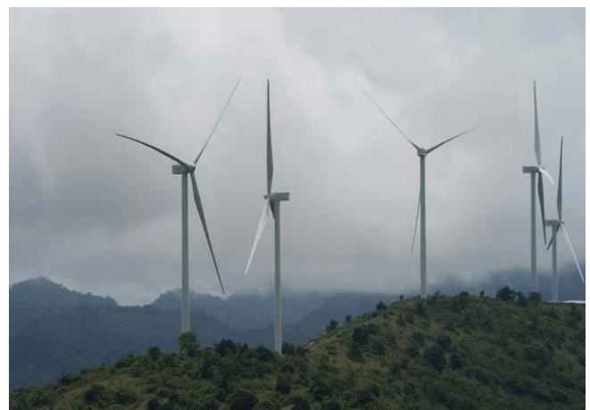
Fig. 1. Tolo Jeneponto Wind Turbine with a capacity of 72 MW
