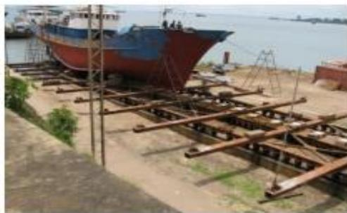
**Gambar 3.** Slipway sistem memanjang (End Launching)
