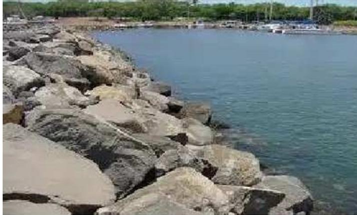
Gambar 1. Breakwater sisi miring
