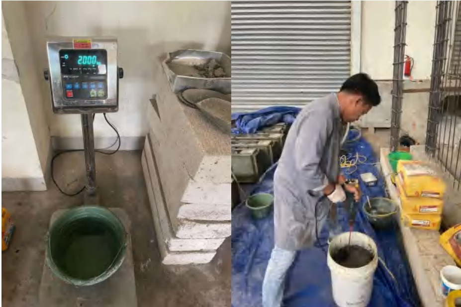
Pengadukan Mortar Grouting
