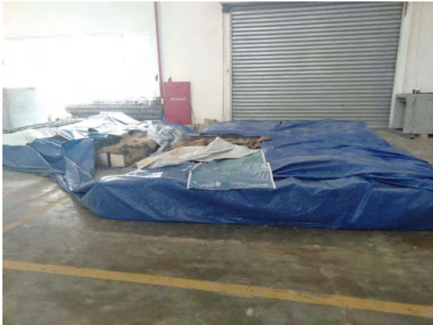
Perawatan Beton/Curing
