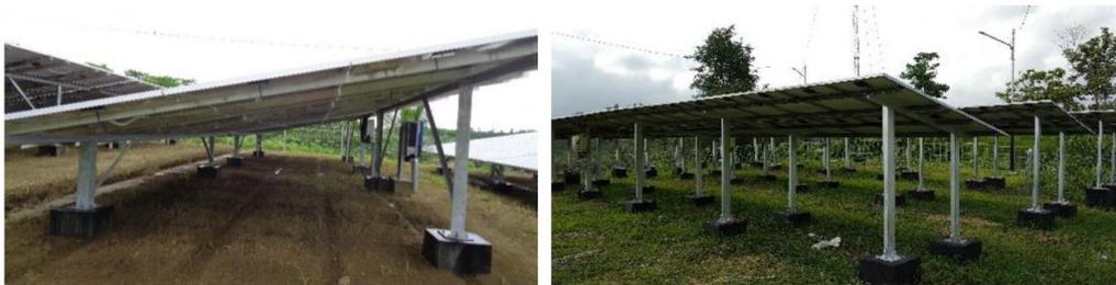
Gambar 16 Contoh instalasi PV ground mounted (KESDM, 2020)
