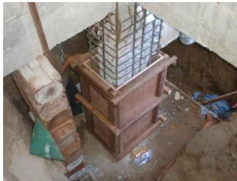
Gambar 13. Metode concrete jacketing (sumber: http://muhammadridhaagusni.blogspot.com )
