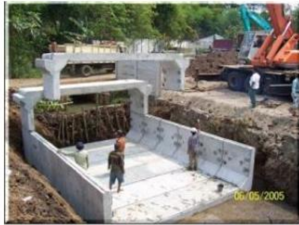
Gambar 2.2 Box Culvert (RCBC)
