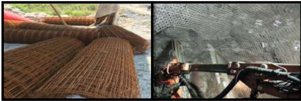
Gambar 2.7 Kawat baja ( wiremesh )
