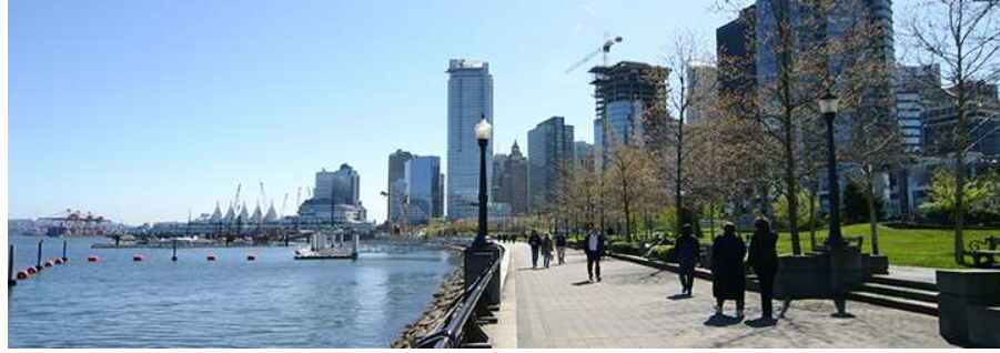
Gambar 2. 5 Vertical Seawall , Vancouver
