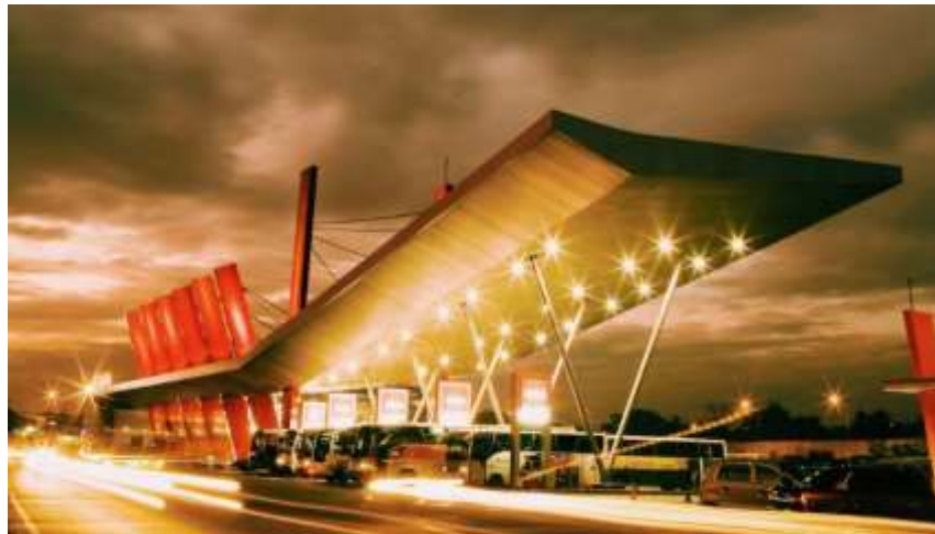
Gambar 2. 12 SPBU Rest Area Tol Cikampek Km 19
