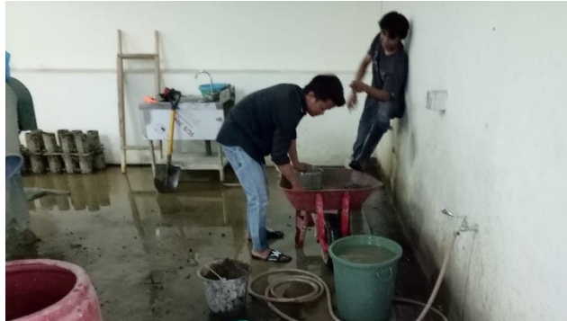
Gambar 6.15 Proses Pencucian Material Beton
