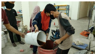
Memasukkan (air + Sikacim Concrete Additive 1%) kedalam campuran
