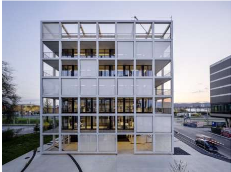
Gambar 2. 1. Tampak bangunan C&P Corporate Headquarters (Sumber: archdaily.com)
