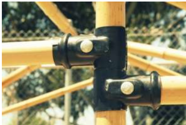
Gambar 7. Sambungan klem/jepit
