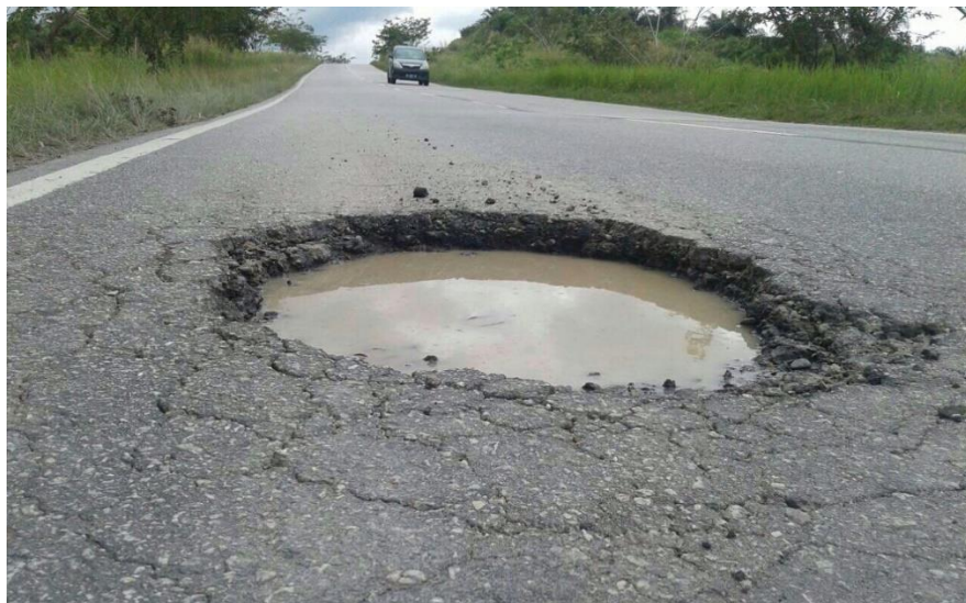
Gambar 2. 9 Lubang (Pothole)
