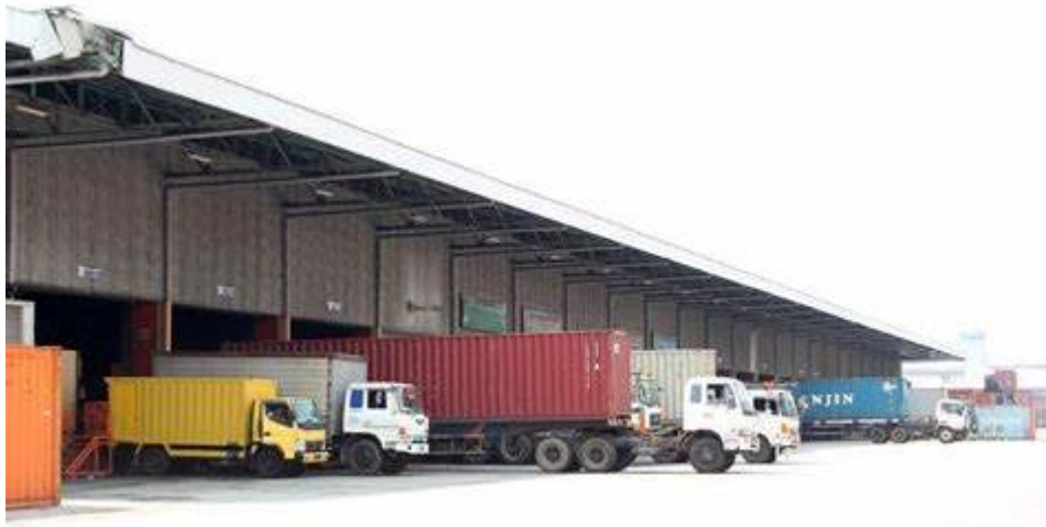
Gambar 2.5 Container Freight Station (CFS)
