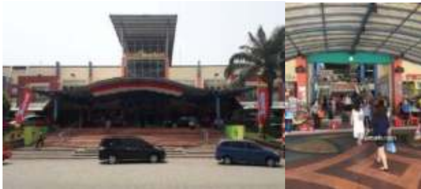
Gambar 2. 20 Tampak Bangunan Frest Market
