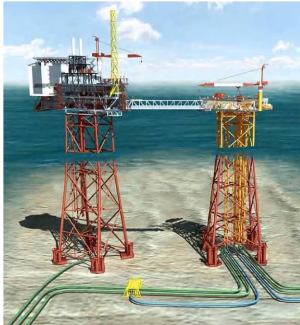
Gambar 2.1 Jacket Platform (Sumber: ramboll.com)
