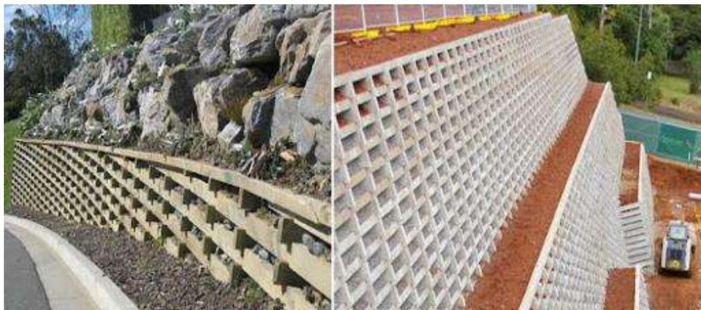
Gambar 9. Dinding penahan tanah *crib walls*
