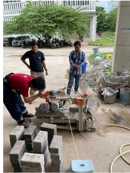
Proses pemotongan paving block
