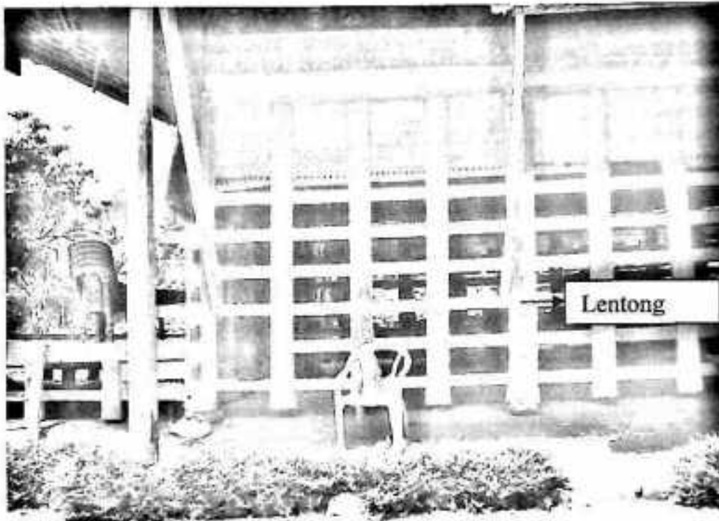
Gambar 4 Tiang penopang lantai (lentong)
