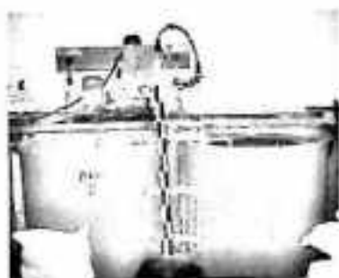
Bak Pelarutan Tawas
