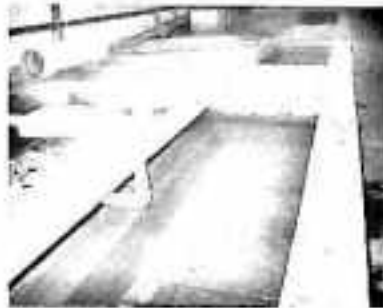
Bak pelarutan tawas
