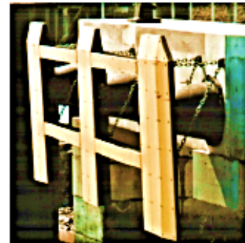
▲ Barry Lock Entrance (WALES)
