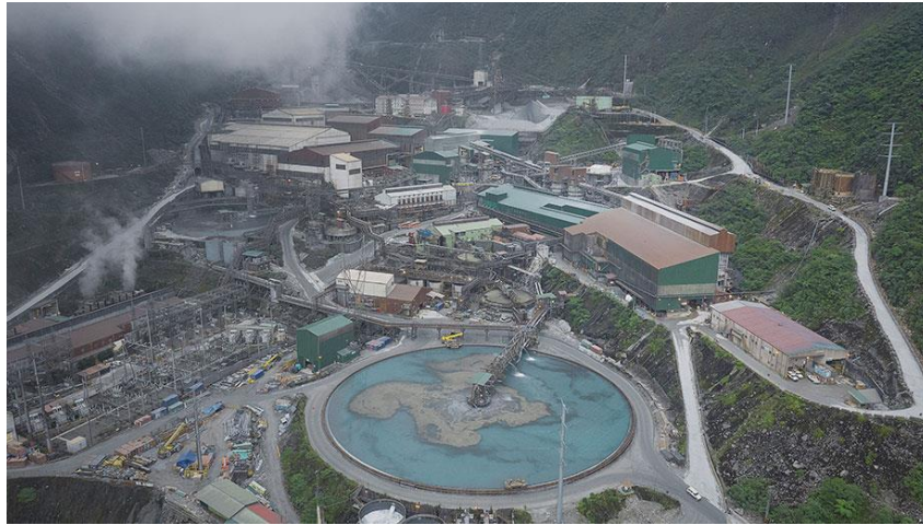
Gambar 2.2: Pabrik Pengolah Bijih ( Sumber: Concentrating Engineering Dept. PTFI, 2016 )
