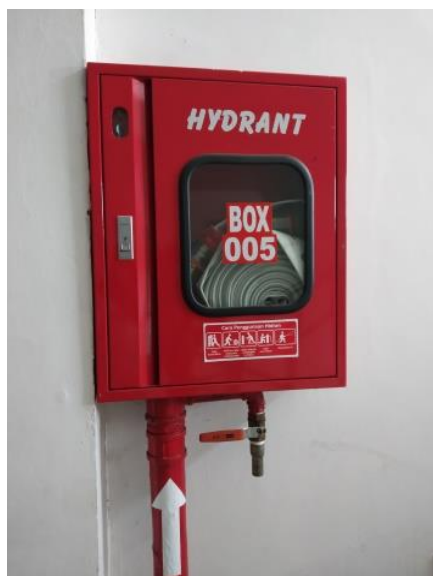
Gambar 2.8 . Hydrant Indoor Sumber: Data Primer, 2020
