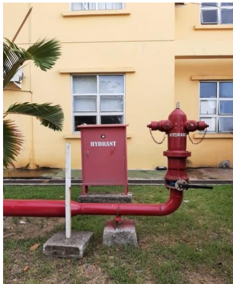
Gambar 2.7 . Hydrant Outdoor Sumber: Data Primer, 2020
