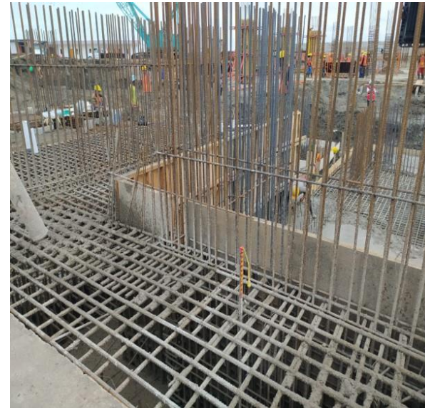
Thermocouple Raft Pondasi
