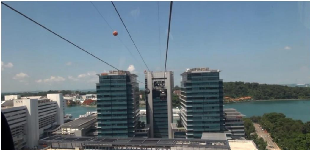
Gambar 2.11 Harbour Front Station Sumber: Yellow Production YouTube Channel, 2013
