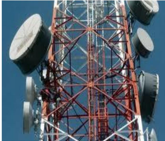
**Gambar 2.13 Antena Microwave**
