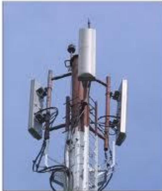
**Gambar 2.12 Antena Sectoral (Grid)**
