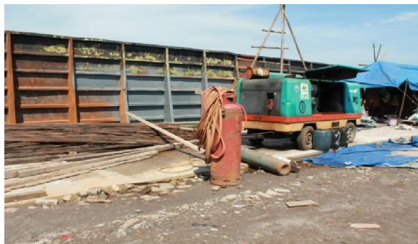
Gambar 1. Persiapan proses sandblasting
