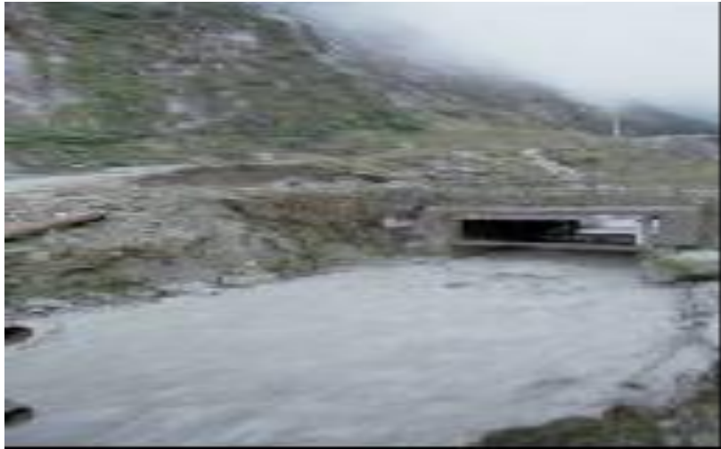
(a) Dam Tailing
