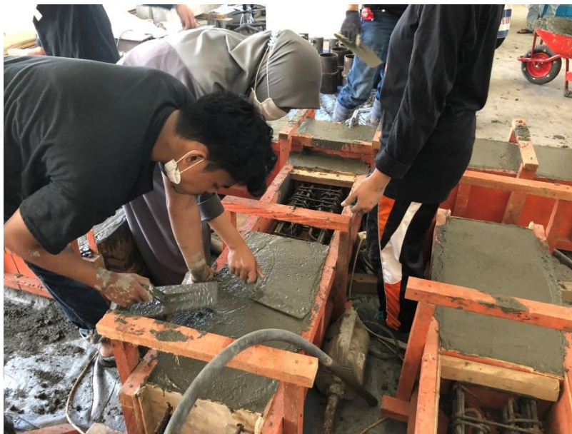
Pengecoran sampel beton BG-1
