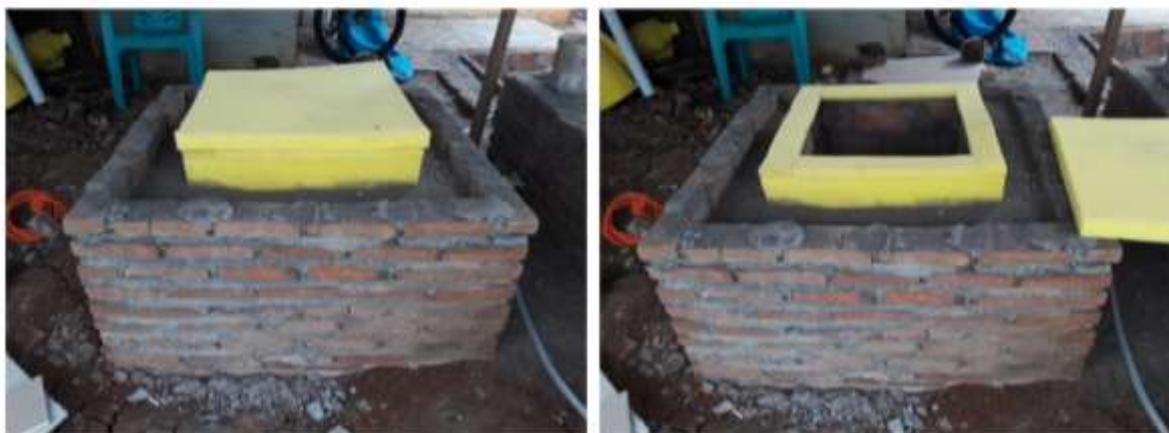
Gambar 2. *Zero Energy Cool Chamber* (ZECC)
