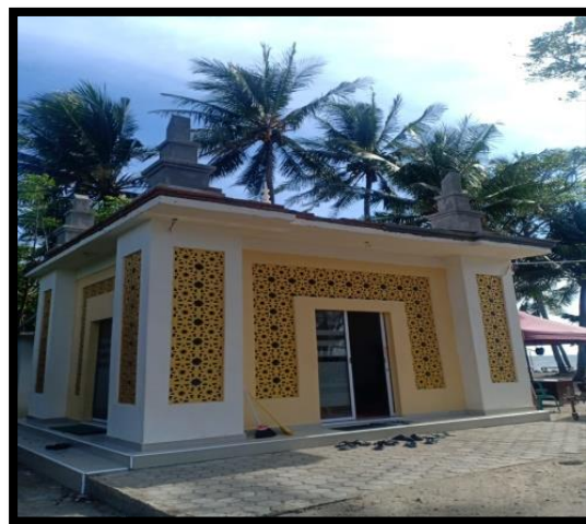
Gambar 22. Kondisi Mushollah Pantai Lawere
