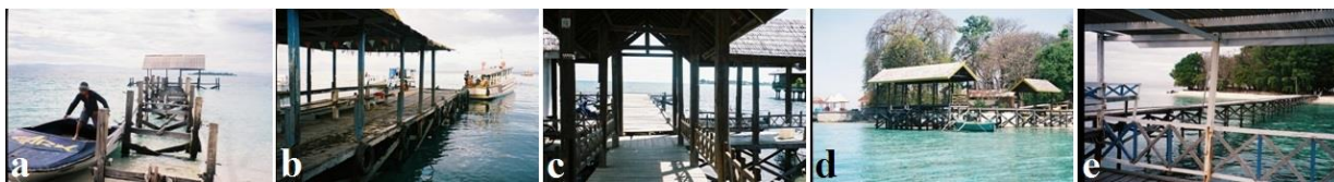
Figure 12. Jetty condition at Langkadea Island, Pangkep Regency (a), Pannambungan Island, Pangkep Regency (b), Barranglompo Island, Makassar City (c-d), and Samalona Island, Makassar City (e)
