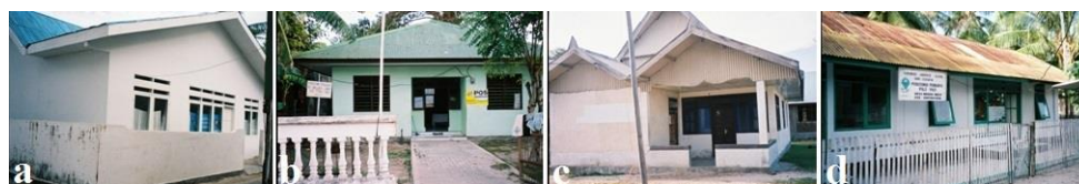
Figure 6. Condition of health facilities at Bonetambu Island, Makassar City (a), Barranglombo Island, Makassar City (b), and Pasi Island, Selayar Regency
