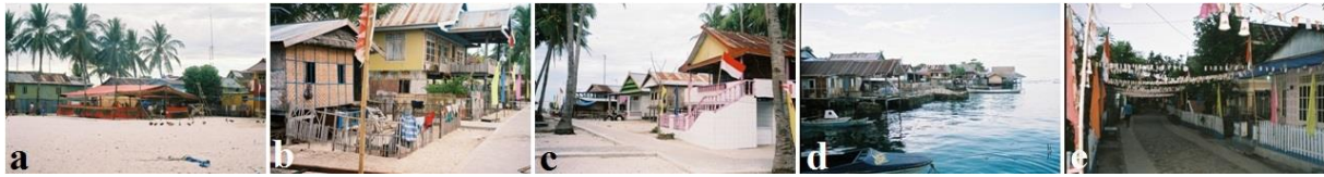
Figure 7. Housing condition at Bonetambung Island, Makassar City (a-c) and Barranglompo Island, Makassar City (d-e)
