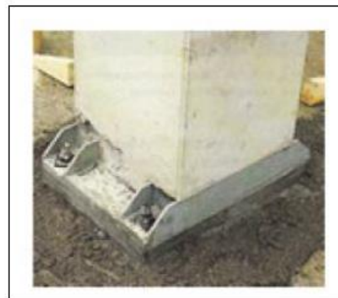
Gambar 2.19. Precast concrete baseplate
