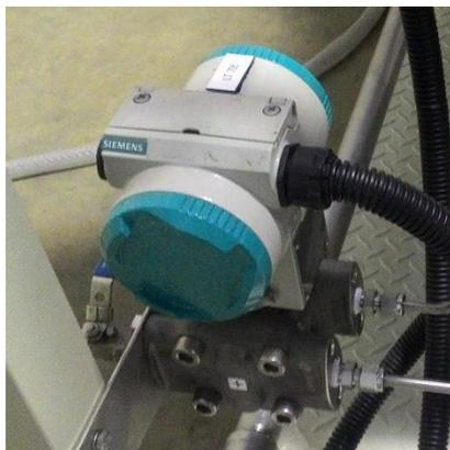
**Gambar 2.15** Water Level Sensor
