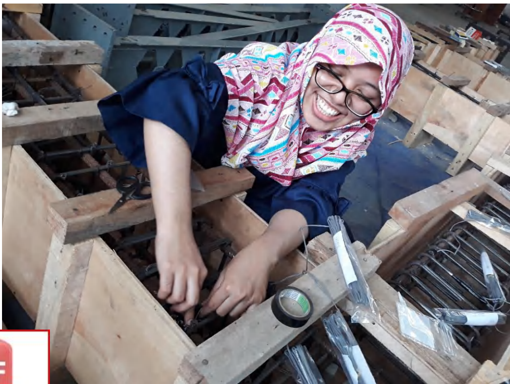
Pemasangan Strain Gauge Sampel Monolit
