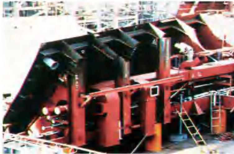
*Gambar 14 Pembangunan Kapal Dengan Aplikasi Integrated Hull Construction, Outfitting and Painting (IHOP)
